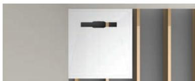
**Step 6.** Final check for former, channel location, waste run and final check of levels for falls to channel. Run a continuous bead of silicone sealant between channel body and former. Drill 3.2mm dia pilot holes 10mm deep max & fix channel body to former using the 8 No 8 x 12mm self-tap screws provided. Do not extend concrete anchor tangs.
