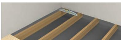
**Step 2a.** Check joist levels are flat and adjust with shims if necessary making allowances. **This is most important as falls on former are shallow for user safety trip reasons.**
