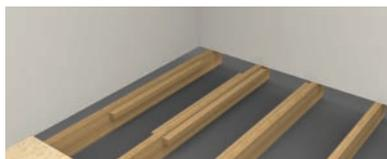
**Step 8.** Attach suitable battens to joists to accommodate flush fitting floor supports.
