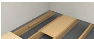
**Step 9.** Cut loose fit floor supports flush to joist top - needed to prevent surrounding floor deflections.
