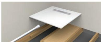
**Step 10.** Connect waste pipe & test for leaks. Connect electrical earth/equi-potential bonding connections to the M8 stud provided if required.
