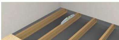
**Step 2b.** Check joist levels and flat both ways and adjust with shims if necessary. **This is most important as falls on former are shallow for user safety trip reasons.**
