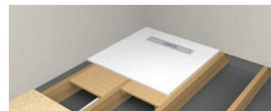
**Step 11.** Slide in floor supports. Do not force past waste pipe or stops moulded on underside of former. Secure former to joists using Ø5 x 50mm countersunk screws on 150mm centres on each joist ensuring former underside is flat and horizontal when installed. Final check on falls to channel See Fig B overleaf.
