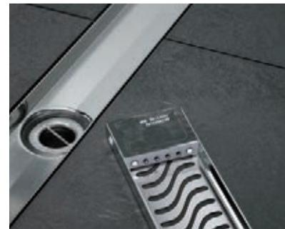
Insert LED units and fix with plastic pins, then re-insert the grating.
